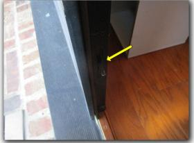
The exterior door frame has some deterioration and/or damage at the sideyard entry door(s).
