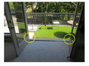
• Water damage and/or deterioration was observed in the wooden exterior balcony entry door(s). This can be a conducive condition for wood-destroying insect activity and/or wood rot.
