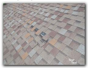
• Damaged drip edge shingles were observed on multiple sides of the roof structure.
