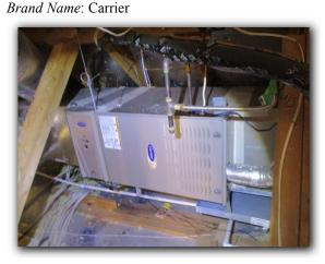
• The indoor blower was observed to be dirty and should be cleaned to help improve the efficiency of the unit.
