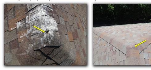
• Any fasteners that penetrate the roof covering should be sealed against water intrusion. The fasteners can be located at, but are not limited to: wall flashing, boot vents, flue vents and shingles.
