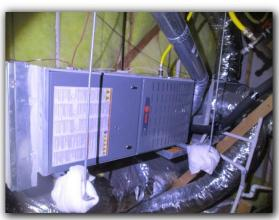
The indoor blower was observed to be dirty and should be cleaned to help improve the efficiency of the unit.
