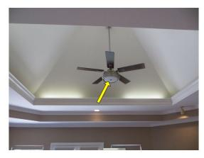
• The ceiling fan is not balanced properly and wobbles when operated in the: upstairs front middle bedroom, upstairs front corner bedroom.
